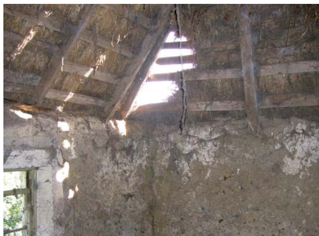
Fig. 16: The roof of this structure of this byre extension incorporates the original hip roof. Note the A-frame structure formed of roughly sawn timber, collar beams and purlins. Again there is no scraw and the thatched is bound to the roof by rope.
