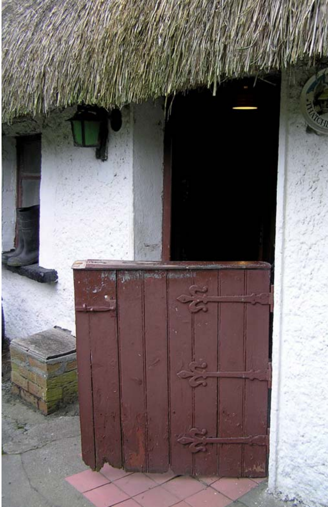
Fig. 28: A half door which is separate from this handsome raised and field-panel led timber front door which leads into a lobby entry house. (Site no. 67)
