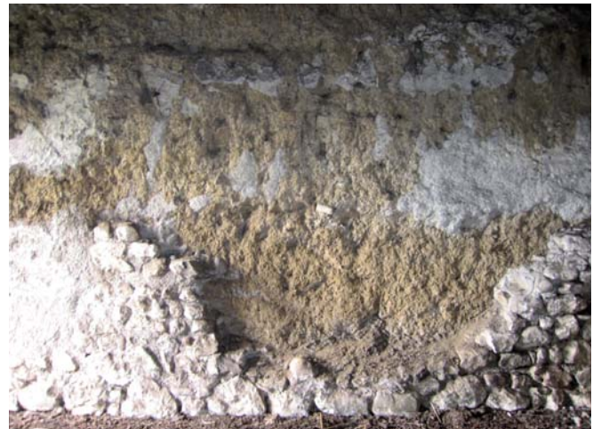
Fig. 21: This clay-walled side elevation has been incorporated within a byre extension. The base of the wall has been built up with a protective layer of rubble stones to prevent damage to the clay wall from animals. The stone facing has partly fallen away taking with it the lime render coating, exposing the clay of the wall.(Site no. 16)
