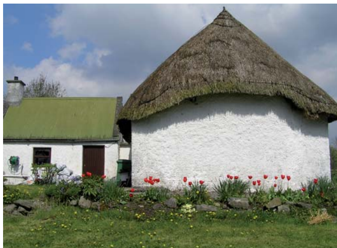
Fig.12: The hipped side elevation of a thatched house in Thomastown has a slight bow resulting in an arc at the eaves . (Site no. 28)
