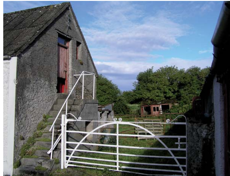
Fig. 30: The relationship between the dairy and the single-storey range of outbuildings proves important in the movement of animals into and out of the farm yard. The wrought-iron gate with characteristic arched brace bar and decorative c-scrolls are typical of these farm gates. (Site no. 75)
