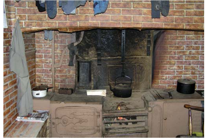
Fig. 27 A traditional hearth with a 19th century range built into the open hearth and incorporating a wrought-iron crane.
