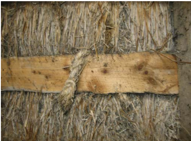
Fig.14: Note the rope used to tie the thatch to the planked purlins. Note also the absence of a scraw. (Site no. 17).
