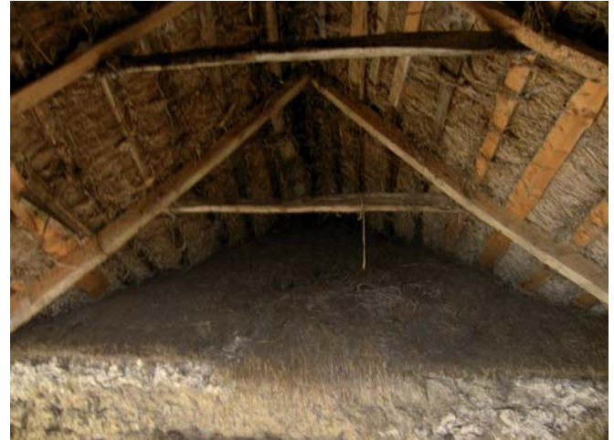
Fig. 15: The byre extension of this clay walled house has a sawn timber roof structure with the thatch placed directly onto purlins, to which it is attached with hemp rope. (Site no. 17)
