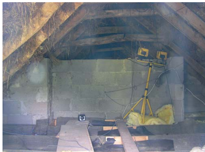
Fig.13: The rough hewn A-framed timber roof structure of example one. (Site no. 24)
