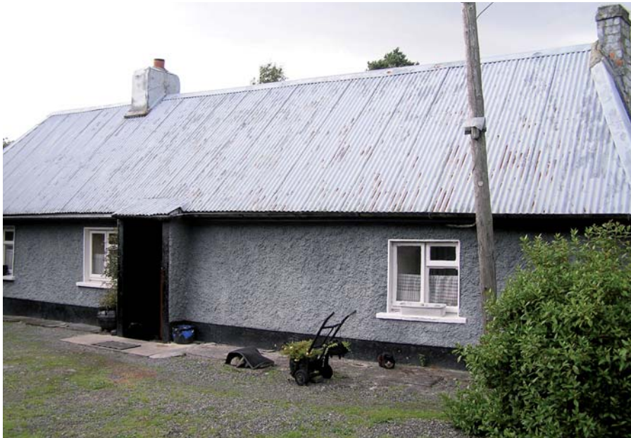
Fig. 19: This tin-roofed structure in Kildoon was put over the existing thatched roof since 1988.
