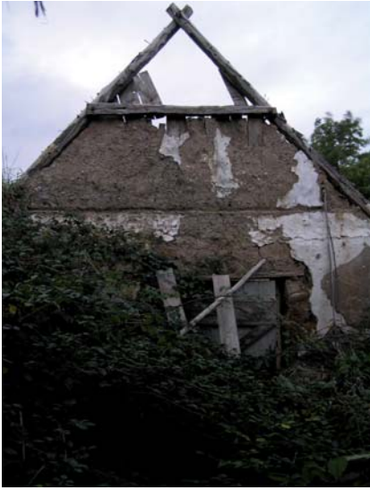
Fig. 26: An internal partition wall, in this case, not a hearth wall, but nonetheless illustrating the incorporation of the A-frame of the roof structure in the wall.)
