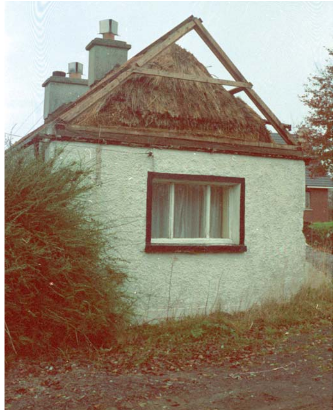
Fig. 20: The tin has been removed from the roof of Silliot Lodge (demolished in 1987), which was located on the road from Kildare to Kildangan. The simple A-frame roof structure was placed over the existing thatched roof. In many cases the chimneystacks have to be built up to take the additional ridge height. (image courtesy of Irish Folklore Department, UCD, A024.09.00049)
